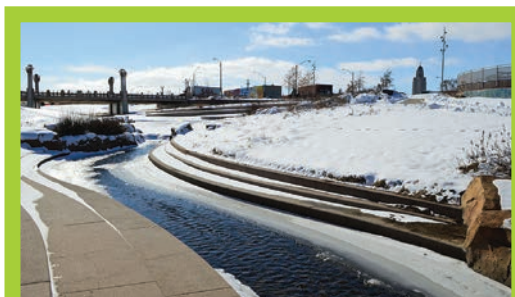
The City of Lincoln built a system to help manage Antelope Creek water flow and prevent flood damage through downtown Lincoln. The project was completed in 2012.
